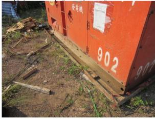
*Photo 3 - A dip tray was provided for the generator that potentially has oil leakage.*
