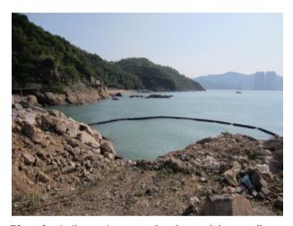
**Photo 2 -** A silt curtain was employed around the seawall area.
